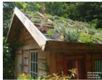
Fig. 2 - Extensive green roof – sloping supporting structure ( www.greenroofromania.blogspot.com )
